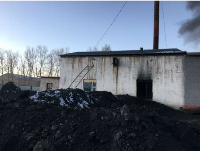
Central heating plant
