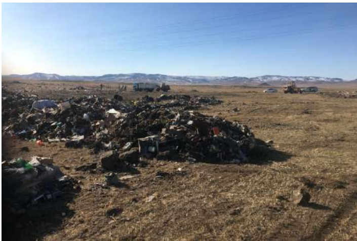
Dumpsite reduction work by contracted private company
