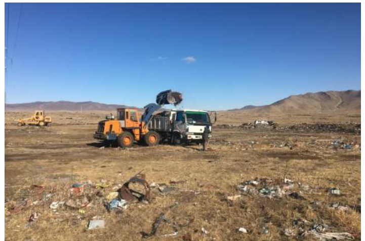
Dumpsite reduction work by contracted private company
