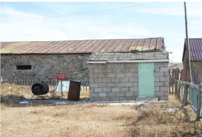
Hospital's waste storage area
