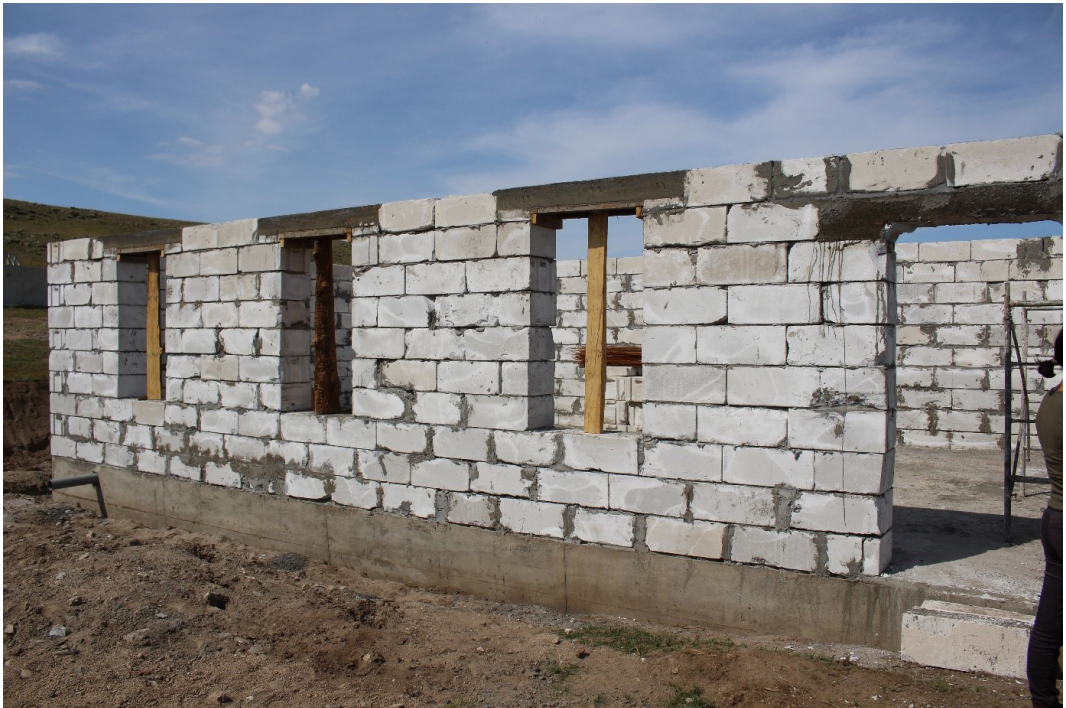
Photo 5. Under construction Waste Management Facility in KU
