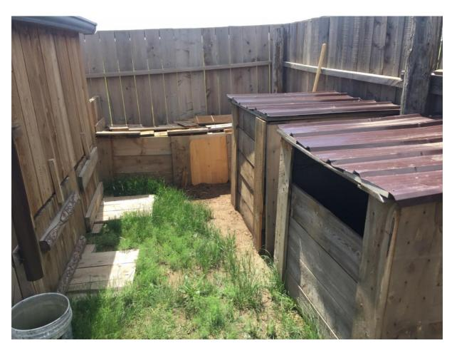
Dry toilets **composting boxes** (which can also be used for organic waste) located right behind toilets
